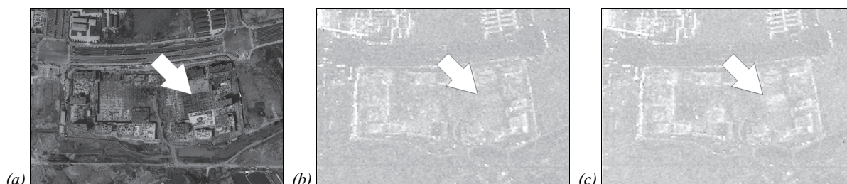
Fig. 2. During the reconstruction that shown in the color image (a) the surface humidity of the region has changed as a result SAR images (b, c) have different brightness
